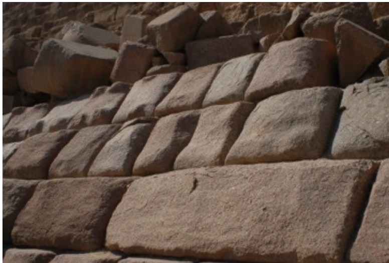
Fig. 5 Casing stones of the Menkaure or Re Pyramid (Note the smooth sides of the blocks in the upper left corner)
