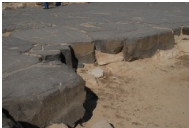
Fig. 7 Cast basalt platform on top of limestone base
