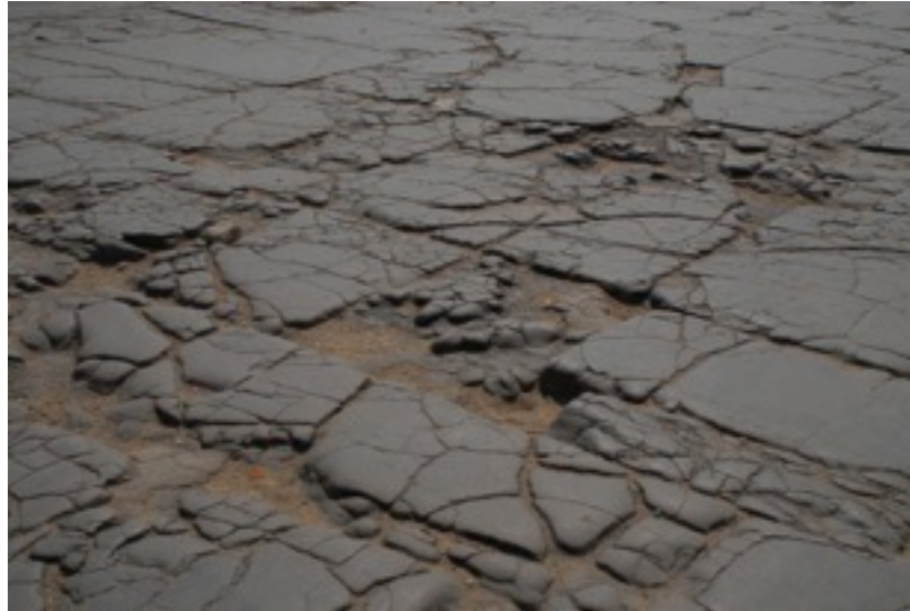
Fig. 6 Basalt platform near the NE corner of the Great Pyramid with cracks due to bad casting
