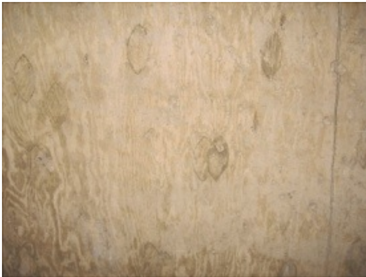
Fig. 9 Plywood knot and wood grain imprints left on today's poured concrete
