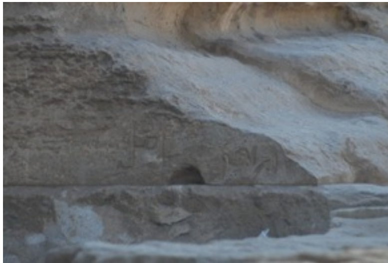
Fig. 4 A casing block on the Osiris Pyramid with an empty casting brace hole
