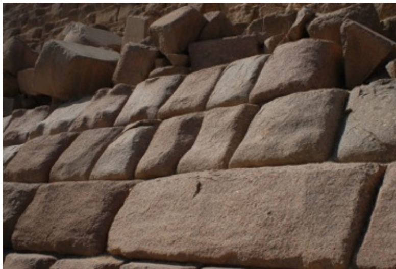
Fig. 5 Casing stones of the Re Pyramid (Note the smooth sides of the blocks in the upper left corner)
